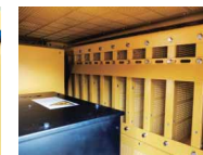
Perforated plate and rock wool within canopy
